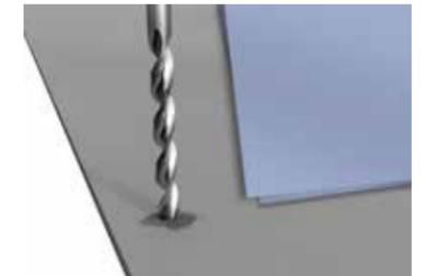
The boards should be pre-drilled with an appropriate fibre cement drill bit. Dust from cutting or drilling must be removed with a brush or a fiber cloth immediately after the work has been completed, otherwise it can mark the surface of the boards.
