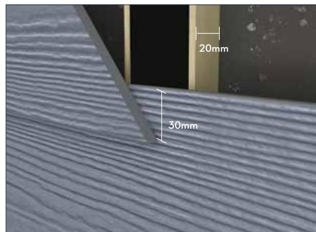
For fast, easy and accurate installation, we recommend using a Cembrit Gecko Gauge. The Geckos assist in creating the correct overlap and ensure the proper location of the screw or nail. Using a Gecko Gauge set clamped to either end of the Planks, makes it possible for one man to install Cembrit Planks.
