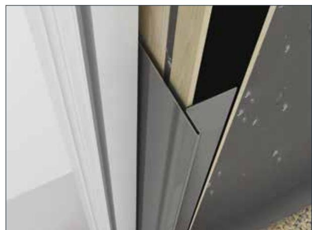
**NOTE!** If using unpainted aluminium in connection with fibre cement products, be aware of surface oxidation.
