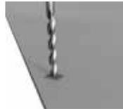
Applying Cembrit Facade Screws. Ensure that the screws are centrally located in pre-drilled holes. Please be careful not to overtighten the screw - especially near the edges and corners of the boards.
